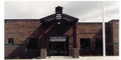
Oquirrh Hills Elementary School – Kearns, Utah
