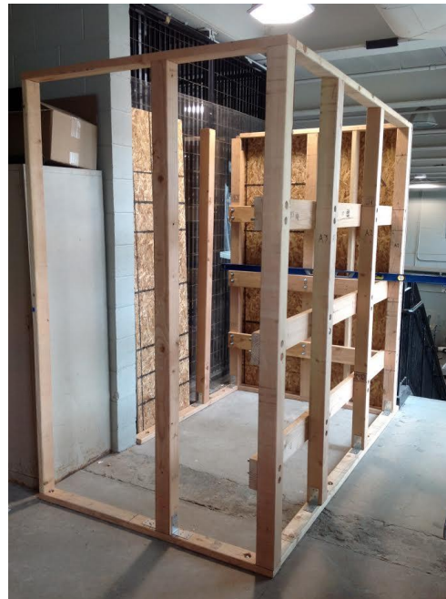
Figure 1: ASR Environmental Chamber during Construction.
