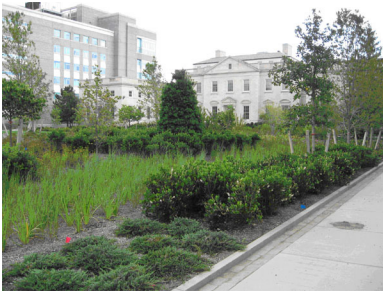
Rain garden plants are selected to tolerate periodic salt conditions and transpire stormwater
