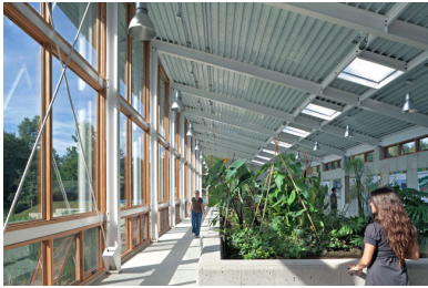
The OCSL has a greenhouse-like atmosphere with solar-tracking skylights and south-facing glazing providing the daylight that the Eco-Machine's water-scrubbing plants need to thrive. Photo © Farshid Assassi
