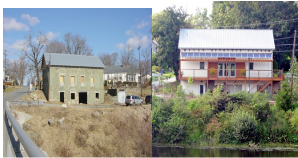
Before and After of the River Resource Center
