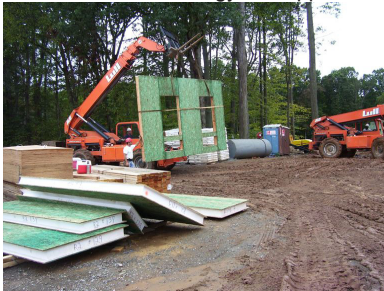
FSC Certified SIPs- Construction Photo
