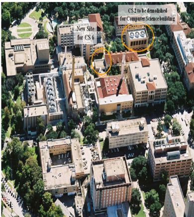
Location of Old Chilling Station 2 and New Chilling Station 6 at University of Texas at Austin
