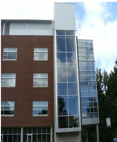
Natural Light Stairwell
