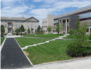
Porous asphalt and bluestone walkways are not intended to be plowed in winter
