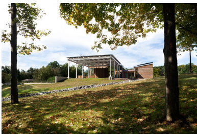
East facade: The restored native landscapes include woodlands, wetlands and prairie. Photo © Farshid Assassi
