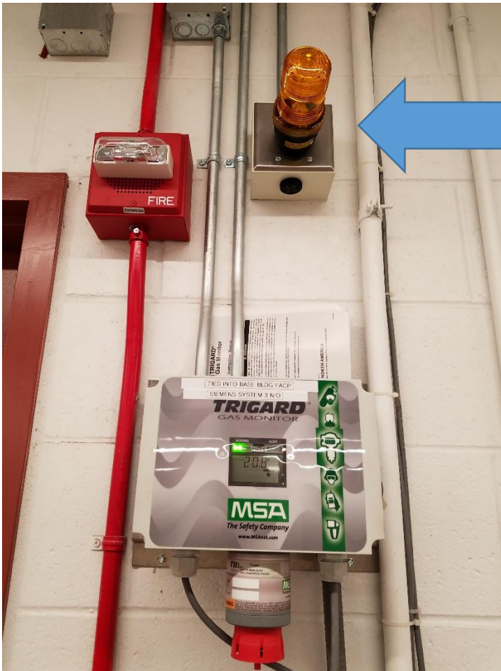
The oxygen monitoring system in normal O 2 operating range
