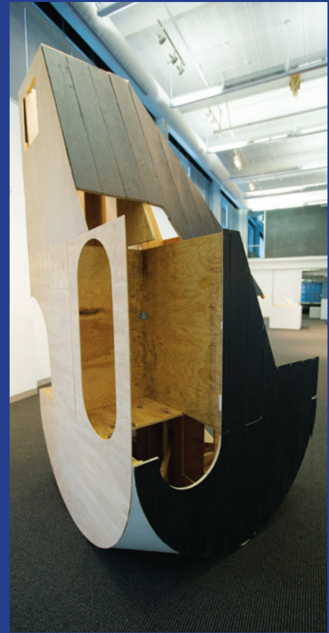
The “Folly,” a 10 ft. by 5 ft. by 5 ft. structure designed by a team of students, that was digitally simulated and fabricated using robotics.
