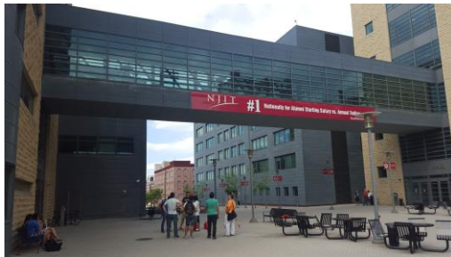
Fig.1 NJIT's steel structure scanned for the research.
