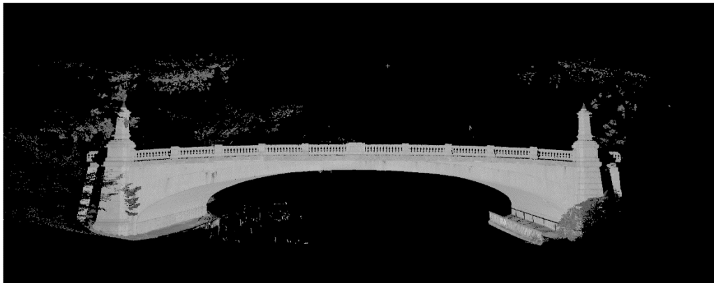
Figure 3 Concrete bridge model created by laser scan as method to identify concrete pathologies
